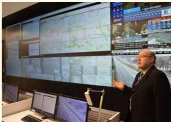
Mississauga is implementing a responsive state-of-the-art Advanced Transportation Management System (ATMS) to manage traffic on its road network. It will allow the City to deal with the increasing traffic volumes and congestion on its roads. ATMS will enable active monitoring of real-time travel conditions, influence the operation of traffic signals, disseminate information and interact with other transportation modes and agencies through the use of hybrid technologies and networks.
