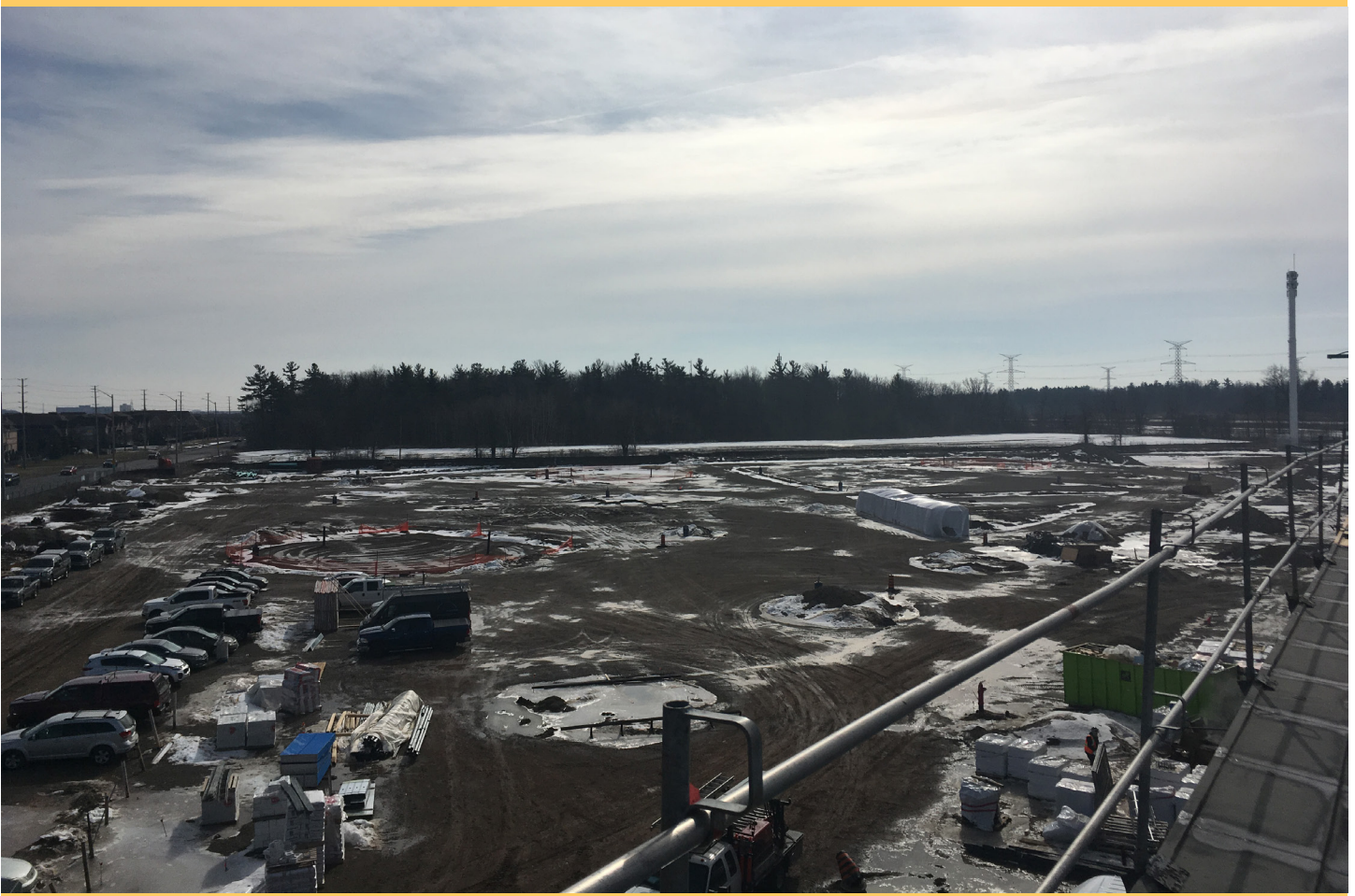
A view from the second floor of the community centre shows the early stages of the parking lot to the south.
