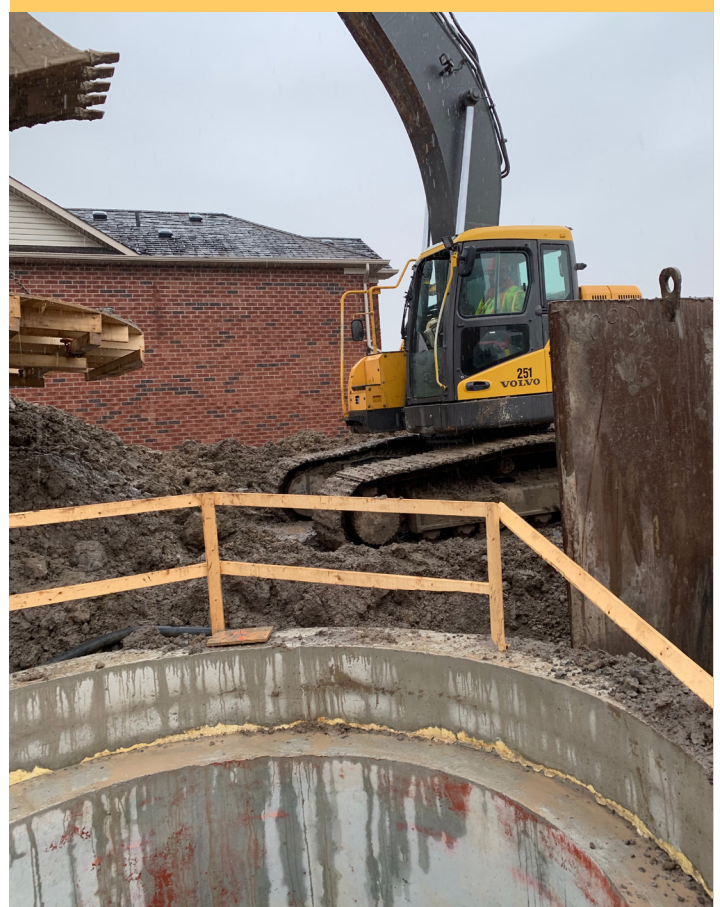
Construction of the Pumping Station at Cactus Gate parkette continues.
